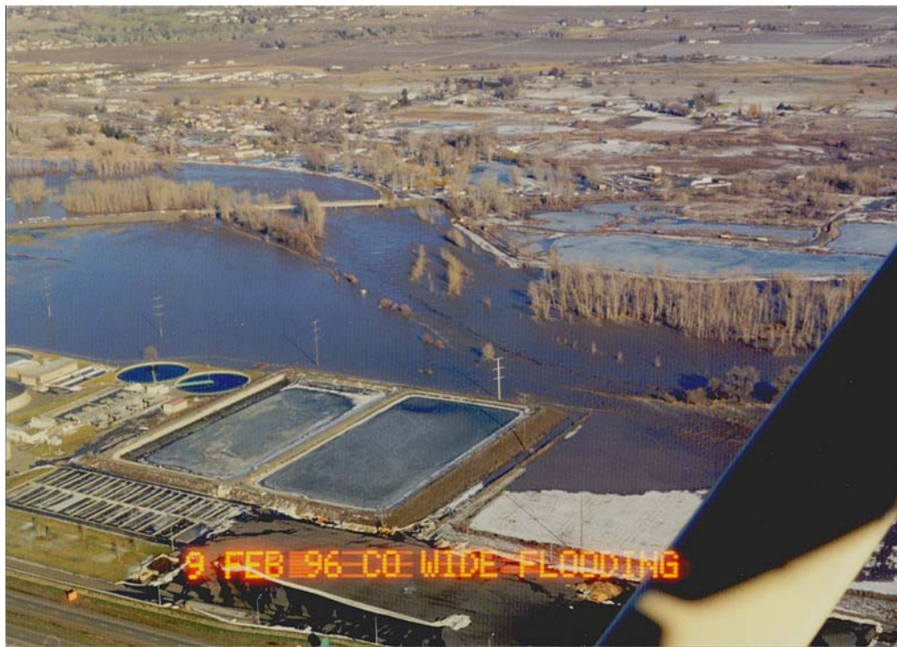
Figure 4-3d. City of Yakima Sewage Treatment Plant, February 1996.
