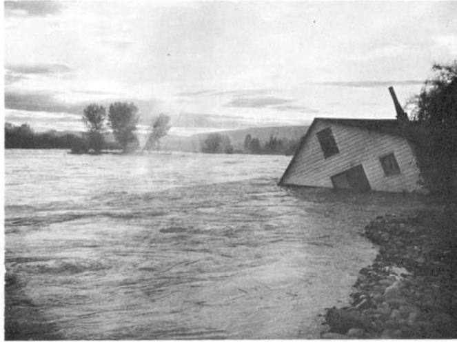
Figure 15.--MAY 1948 FLOOD DAMAGE TO RESIDENCE ON KEYES ROAD
