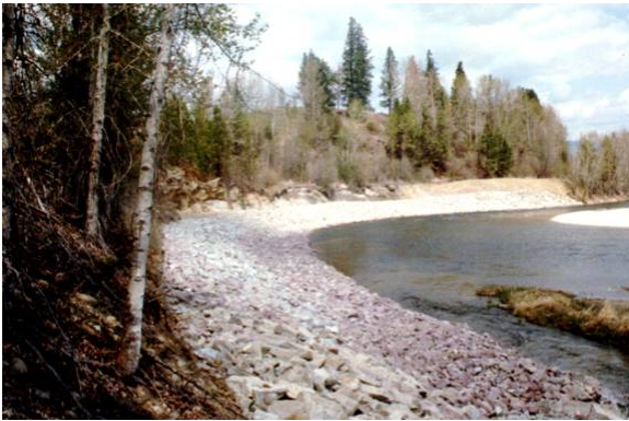
Figure 2.25 ACCEPTABLE riprap for erosion control. (MT)
