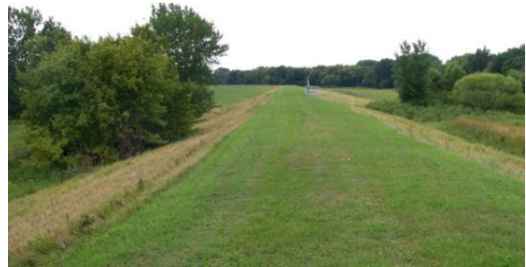
Figure 2.31 UNACCEPTABLE. Levee is mowed but trees and longer grasses within levee easement area. Trees are greater than 2" in diameter. (MN)
