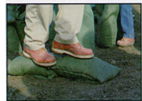
Place each succeeding bag tightly against and partially overlapping the previous one. Compact and shape each bag by walking on it.
