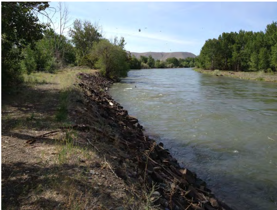
Photo 8: Existing DID #1 levee exposed to direct river attack near Ponds 2 and 3, viewing downstream.
