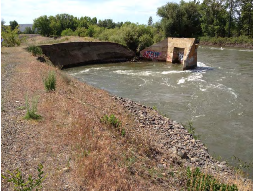
Photo 1: Erosion and undermining at old levee on left bank upstream of SR24 Bridge, viewing downstream.
