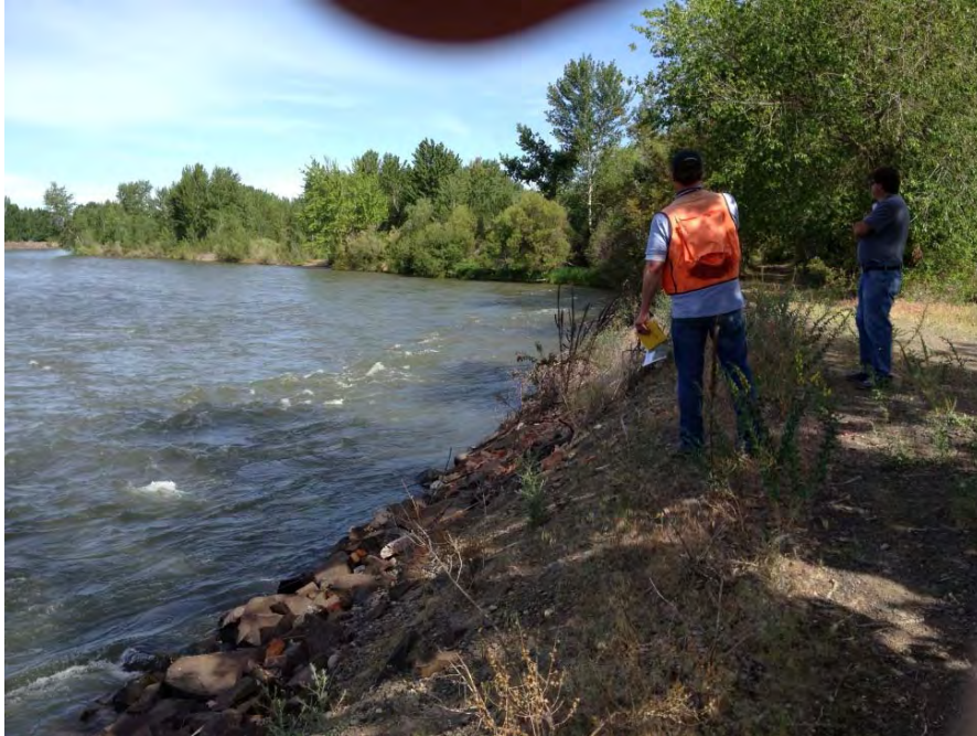
Photo 7: Existing DID #1 levee exposed to direct river attack near Ponds 2 and 3, viewing upstream.
