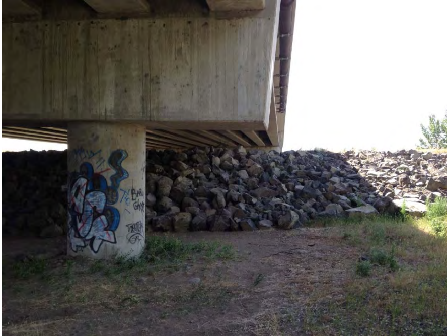
Photo 3: Near left bank at SR24 Bridge showing cross-dike blocking floodplain.
