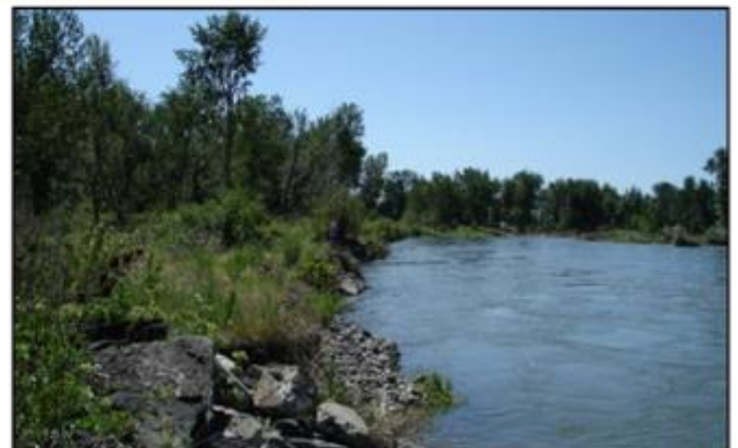
Concrete debris to be removed
