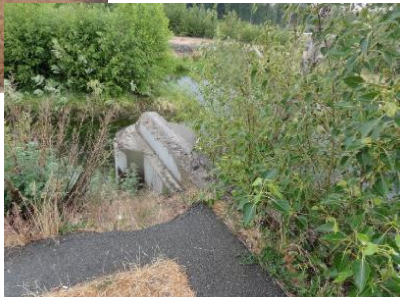
Abutment for Removal
