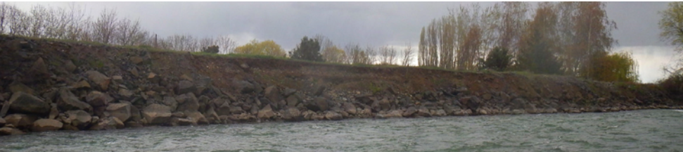
Failing revetment along avulsion path near RM 8.6.
