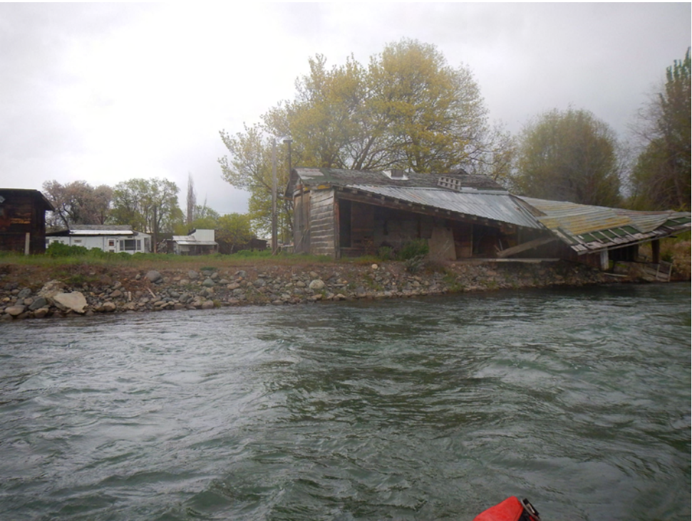
Lateral meander migration destroying an abandoned structure at RM 8.3.
