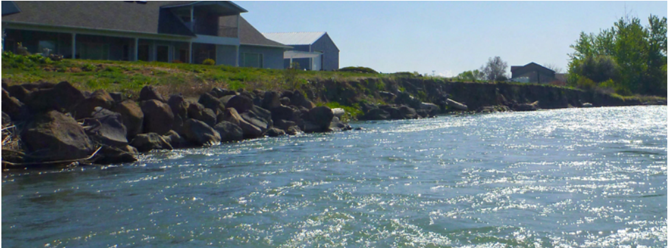
Left bank Erosion at RM 7.85 threatens homes. Erosion is into 1st terrace above geomorphic floodplain and mobilizing relatively abundant fines.
