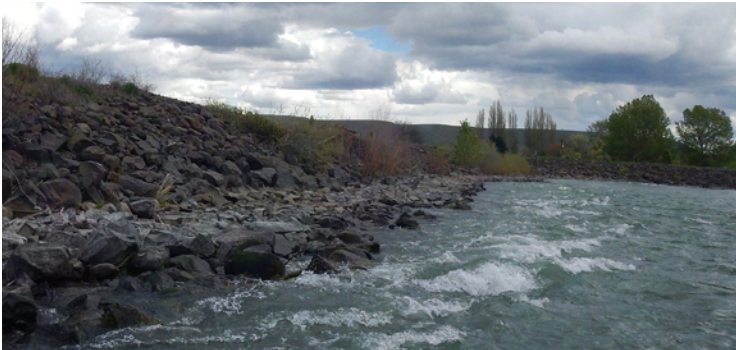
Thalweg held against upstream portion of N7 levee near RM 14.0.
