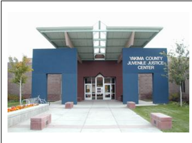
1728 Jerome Avenue, Yakima, WA
